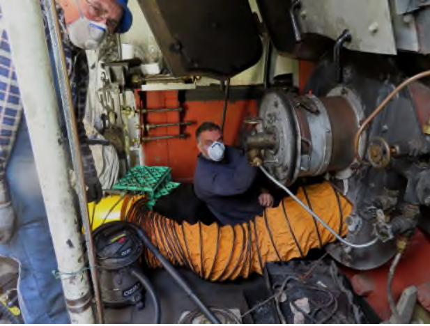
Alex and Derek cleaning lower boiler, Jan 2021
