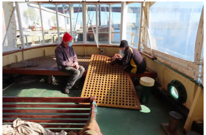
Ian and Ken cutting exhaust pipe space for generator, July 2021
