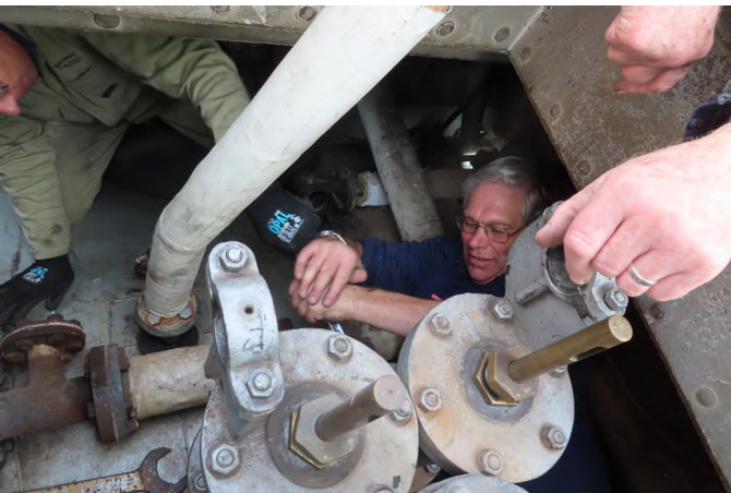
Richard working on safety valve on top of boiler, March 2021
