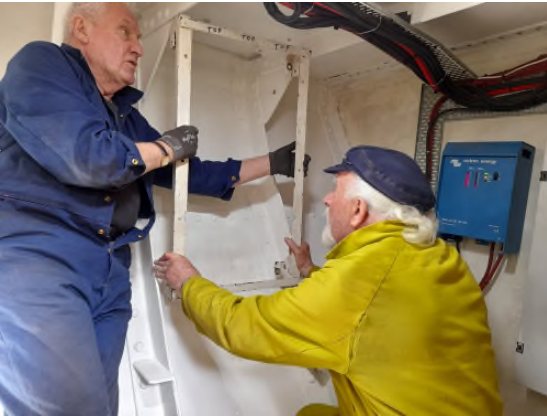
Bruce and Wally refitting old switchboard frame, May 2021
