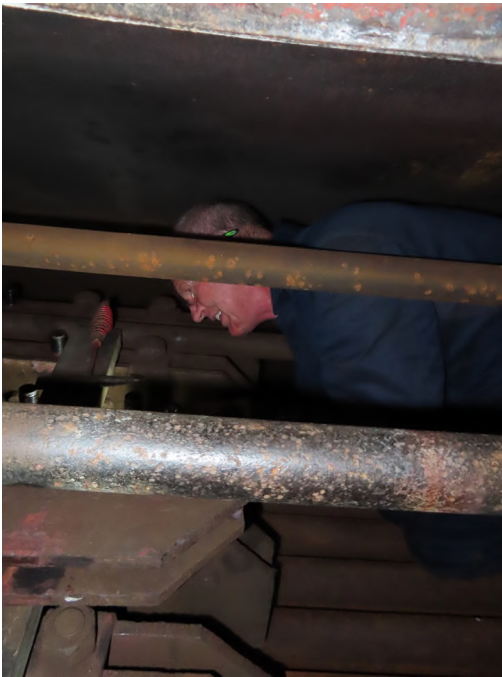
Tim inside boiler, Dec 2021
