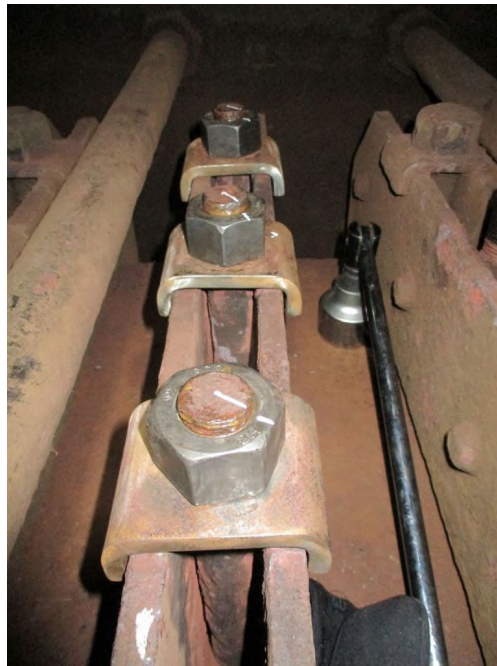
Retainers and nuts replaced and tightened, Dec 2021
