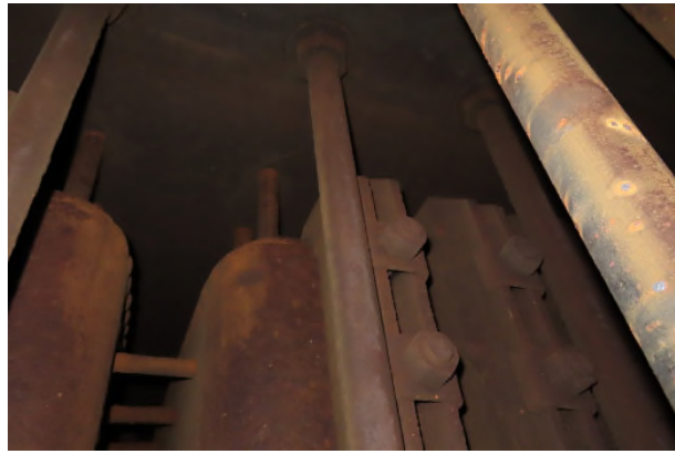
Looking inside the boiler after cleaning
