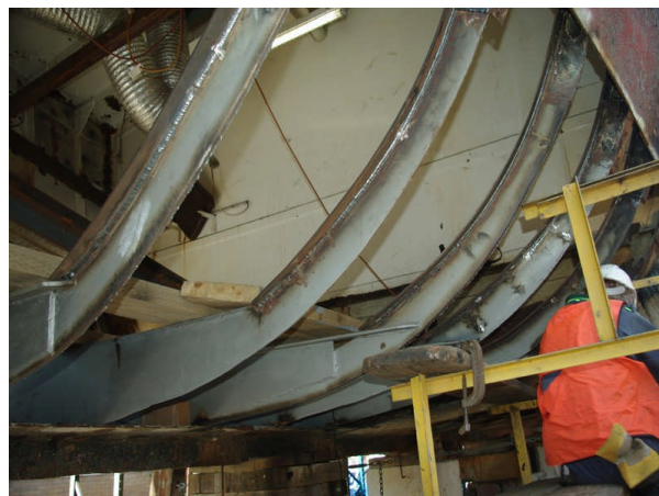
Flanges welded to inside of frames
